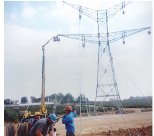
Controlled cable tensioning
